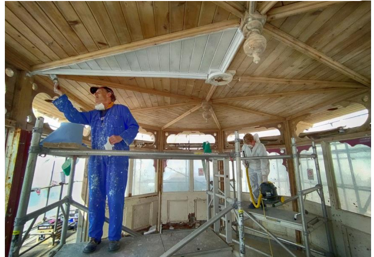
The first lick of paint goes on the Bandstand.
