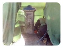
Our first step was to seek help from a local specialist called Blasted Bare who prepared the surface by removing all the old paint, rust and grime through sandblasting.
